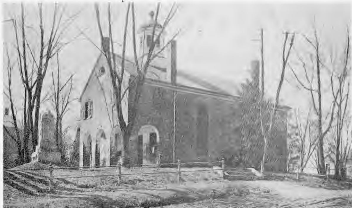
THIRD FAIRFAX COURT HOUSE, BUILT IN 1800. MONUMENT IN FOREGROUND INDICATES SPOT WHERE FIRST SOLDIER WAS KILLED IN BATTLE DURING THE CIVIL WAR.
