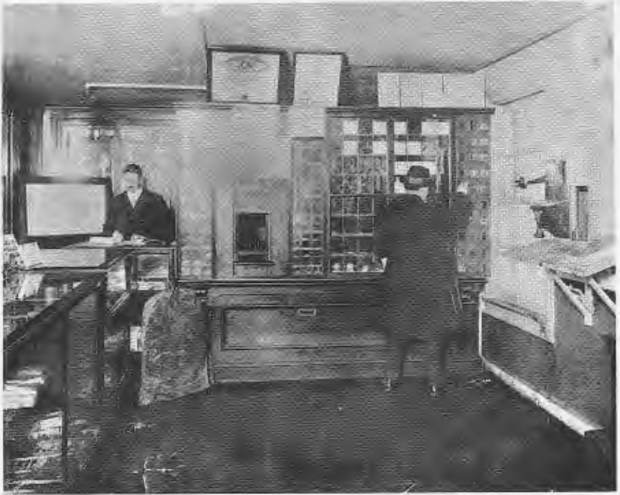
Combination Ballston Pharmacy, Post Office and Railroad Waiting Room
