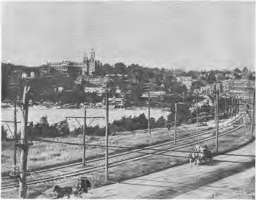
The electric railway tracks in Rosslyn, overlooking Georgetown.
