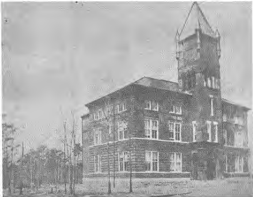
The 1898 Courthouse as it looked the year it was built.
