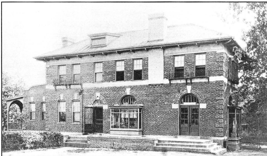
From the collection of Kathryn Fearson Chesapeake and Potomac Telephone Company Building at the intersection of North Irving Street and Clarendon Circle, circa 1921.
