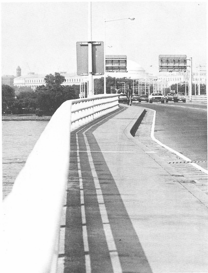
The current span. Photo by James Barron.
