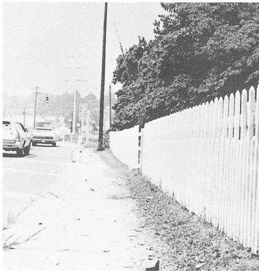
The same site, including the fence, 1973. Photo by James Barron.
