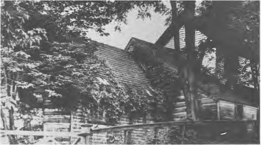
The Ball-Sellers House about 1908 showing the kitchen wing which was torn down in 1915
