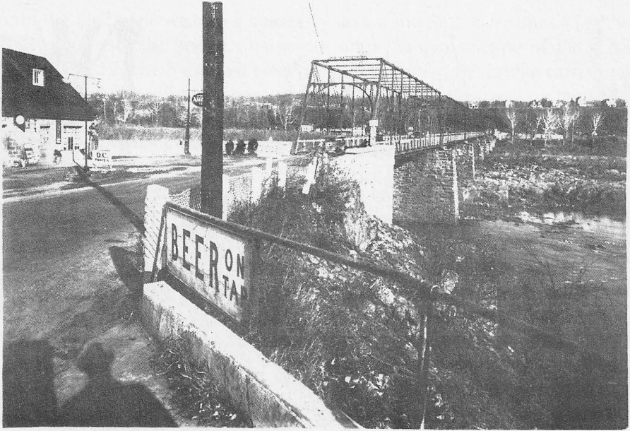
Virginia end of bridge — Circa 1930. 1927 abutment visible. Picture taken from Mackey Tavern parking lot. Courtesy Commission of Fine Arts, Donald Myer
