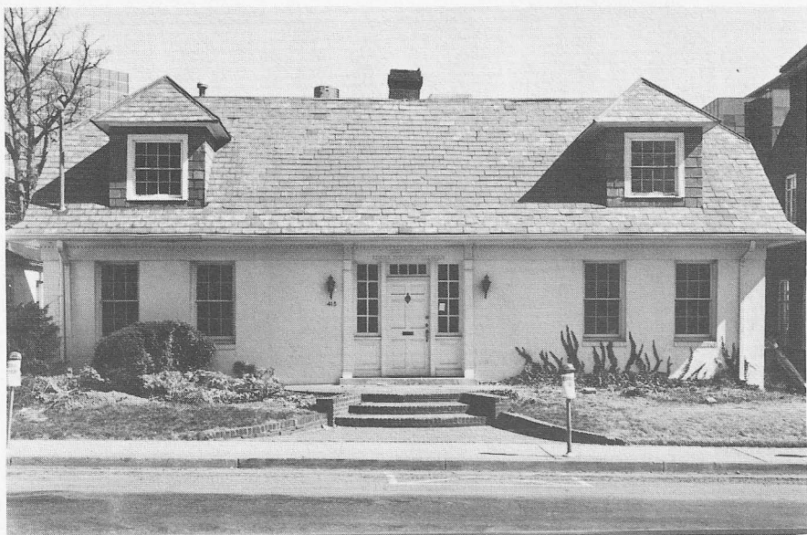
Moncure Building (Adams, Porter, and Radigan Building), 1415 N. Court House Road SCHWARTZ
