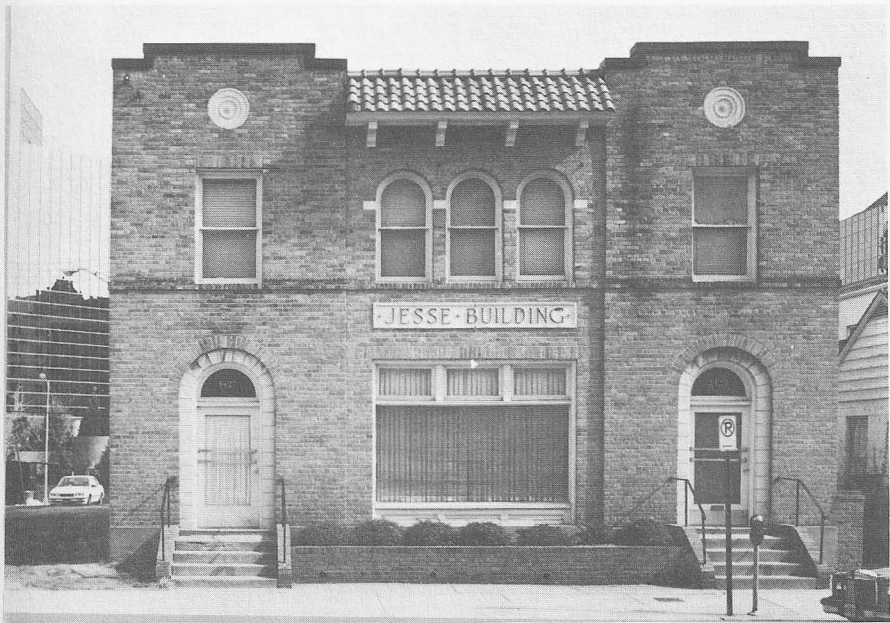
Jesse Building, 1423-27 N. Court House Road
