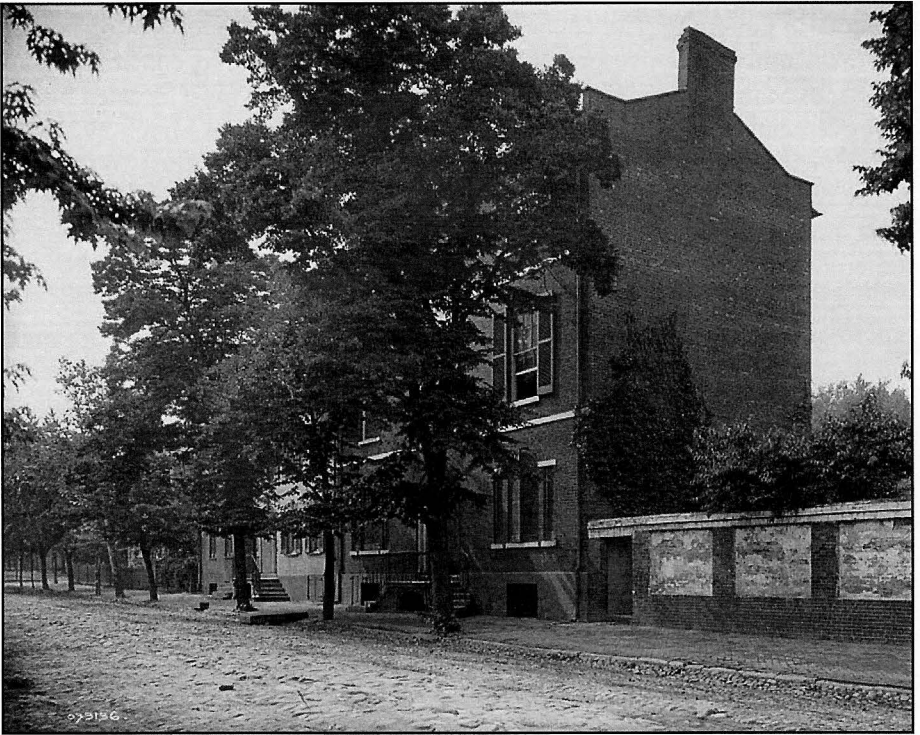
Figure 3. Wheel ruts and other damage to the cobblestone pavement are visible in this picture of Cameron Street in Old Town Alexandria. Maintenance eventually became too costly for the city, which decided to discontinue repairs on cobblestone roads in the late nineteenth century.
