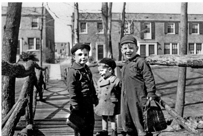
Fig. 2: Arlington Village at Bridge Across H-Court Hill
